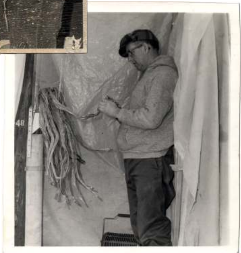
A newspaper article which accompanied this photo states: "SPLICER AT WORK - A big part of the work involved in changing the Dashwood exchange of the Hay Municipal Telephone System to dial is the endless amount of cable splicing required. Shown here at the tedious job is Jack Keller, of Seaforth, who does most of the splicing for the Hay System. He works inside a tarpaulin hut, with a small propane heater helping to keep his fingers warm. Dashwood residents will be seeing quite a bit of this hut over the next few weeks." .....
