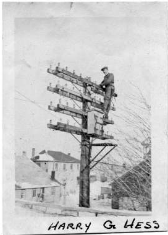
Harry G. Hess up a 4 – 10 pin cross arm telephone pole in the early 1900’s.
