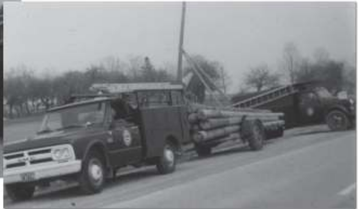
Lloyd Denomme directs a telephone pole that is being hoisted off the trailer by the line truck. It is then guided into the previously dug hole.
