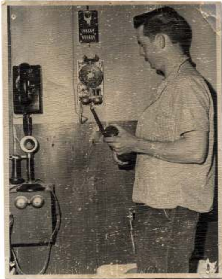
This now well aged photo from the mid 60's was used in a newspaper article showing Lloyd Denomme installing a new fire alarm telephone on the premises of Fire Chief Milton Deitz. Above the phone is a switch to turn on the fire siren when a fire call was received on the special telephone. Below the new phone is the old style set that was in use for years. .....
