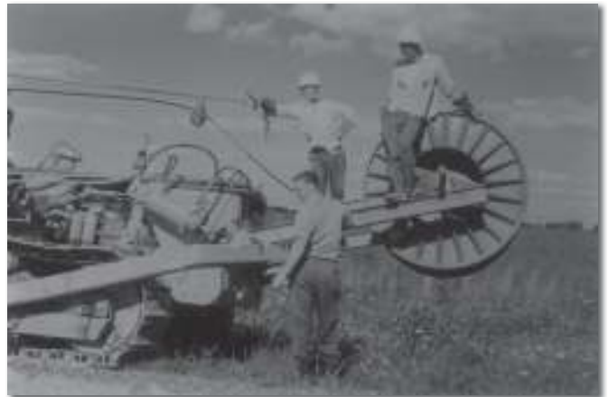
From the top left, Gerry Chapman and Ivan Meidinger stand on the cable plow and Doug Armstrong stands on the ground.
