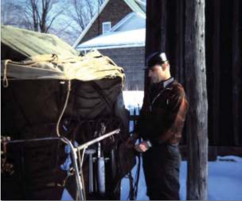
Steve Meidinger in 1964 splicing underground copper cable preparing for the Zurich cut-over.
