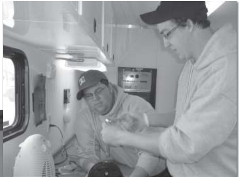
In 2010 fibre to the community and to the home was initiated. Shown here, Dan Drennan, left and Matt Janmaat assemble the fibre splice case prepping for the splice. They are in the new environmentally controlled fibre trailer where highly precise fibre splices are completed.
