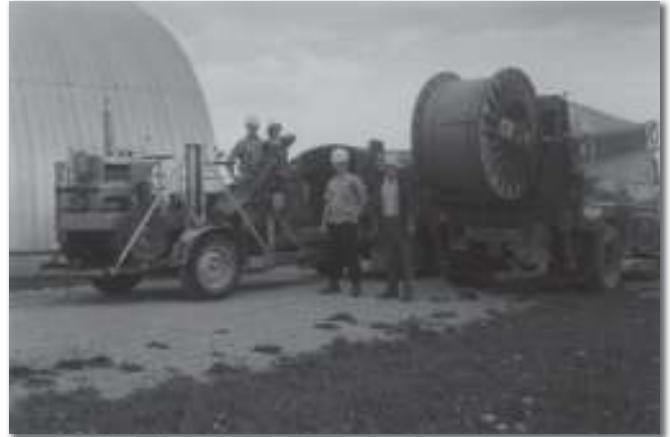
This 1960’s photo was taken by the Quonset hut in the yard at Hay with the line truck and a trencher. Shown from the left are Steve Meidinger, Jack Keller, Doug Armstrong and Gerry Chapman.
