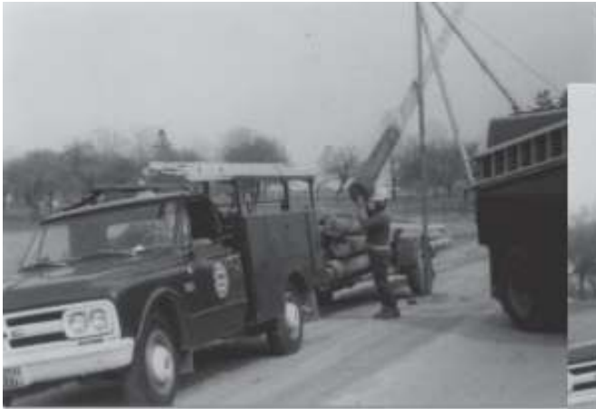
Lloyd Denomme directs a telephone pole that is being hoisted off the trailer by the line truck. It is then guided into the previously dug hole.
