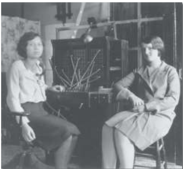
Rosella Krueger, left and Lottie Gascho at the Zurich switchboard. .....
