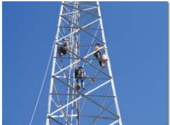
2009 - Construction workers inside the new wireless internet tower in Mt. Carmel. The equipment will service customers outside of Hay's traditional coverage area as many of these customers are still on dial-up internet service.
