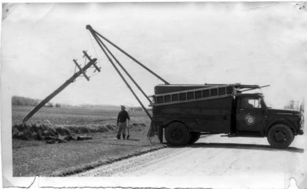
Also from the Citizen, "Miles and miles of telephone lines in the Hay Municipal System were broken down by the unseasonable sleet and wind storm throughout this area last Wednesday.... Shown here is line foreman Harold Zehr supervising the replacement of a broken pole, as fellow workman Stephen Meidinger operates the truck hoist. This activity was taking place on the Bronson Line north, in Hay Township. (Citizens News Photo)"
