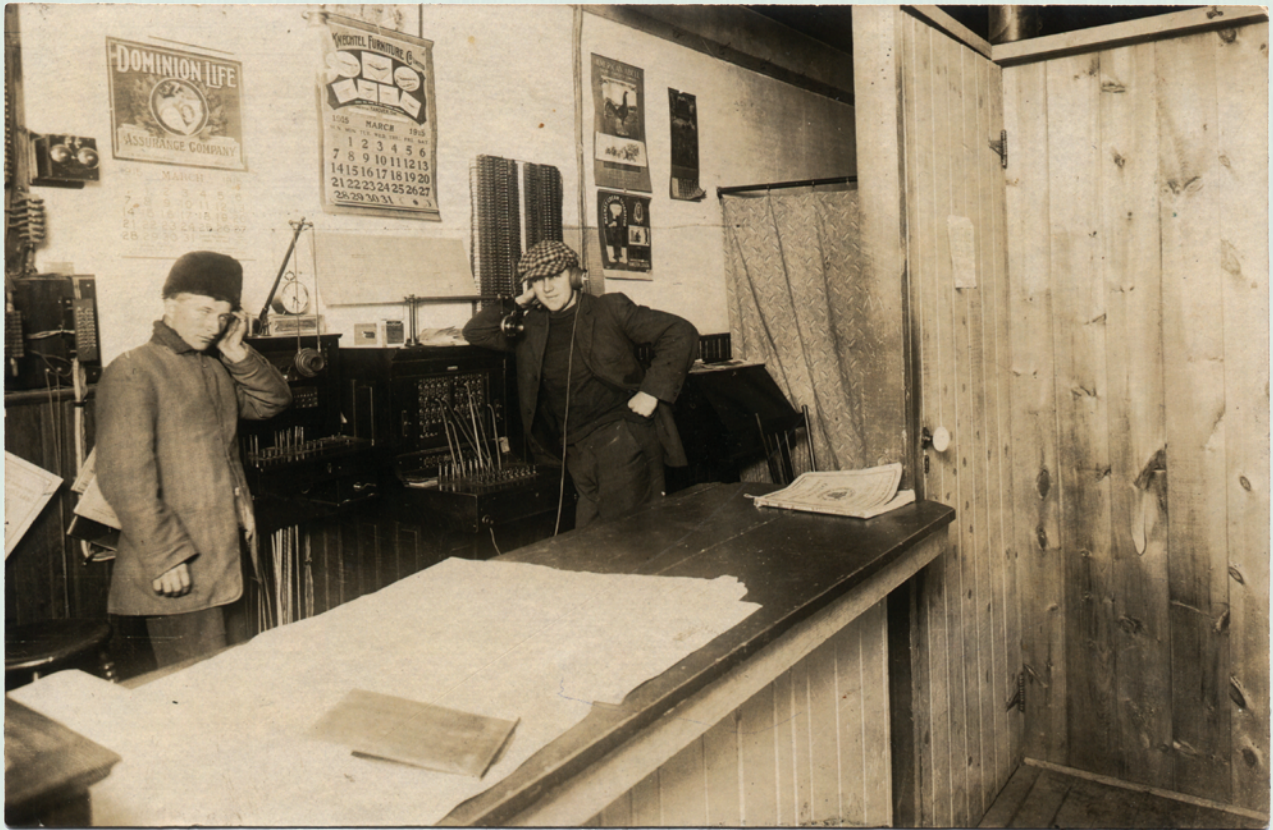
"Bobby" Willert, left and Irvine McIsaac working the Dashwood telephone switchboard in 1915. The switchboard was located in the front part of Tieman's Furniture Store.
