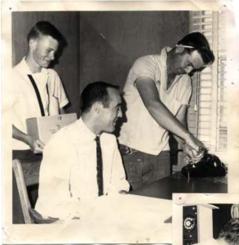
This photo taken in 1966 shows a magneto to dial conversion at the Bank of Montreal in Dashwood. Lloyd Denomme is the installer, Peter Regier is the installer's helper and the accountant from the bank is unknown. .....
